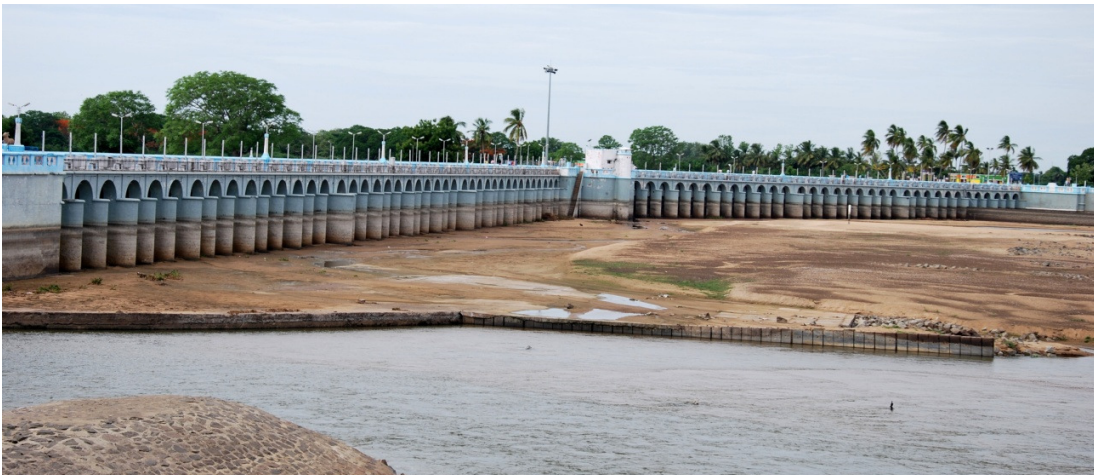
The 329-metre-long ‘Grand Anicut’ ( Kallanai in Tamil) across the Kāveri River, thought to have been constructed by the Chola king Karikāla some 1,800 years ago (it has been restored several times since), is a massive and effective water-diverting device, splitting the river into four streams and irrigating thousands of hectares of agricultural land in the Kāveri delta. (Courtesy: Michel Danino)
